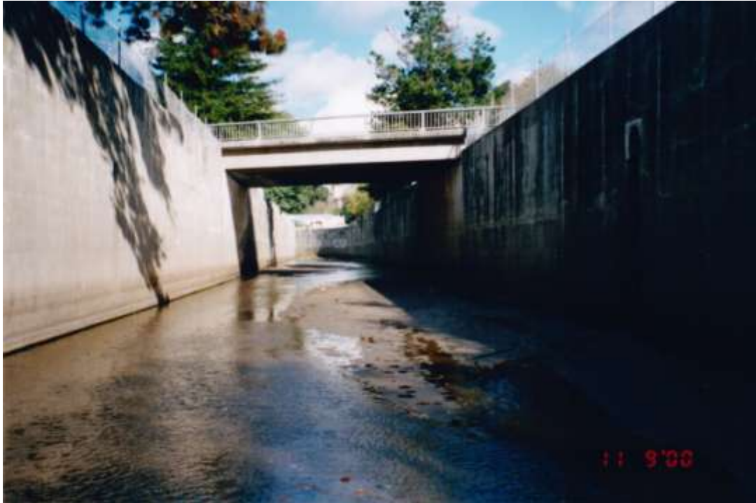
Branciforte Creek Flood Control Channel
