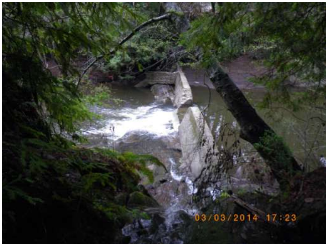
Barker Dam on the middle mainstem San Lorenzo River– Reach 9 (below Boulder Creek confluence at Spring Creek confluence).
