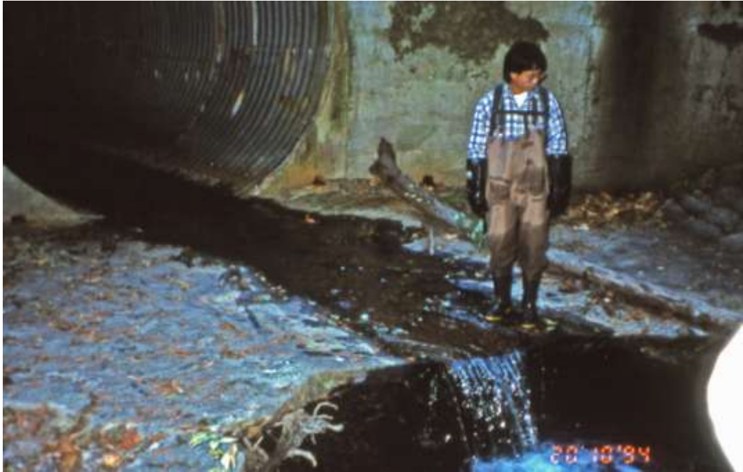
Highway 9 Culvert and Concrete Apron at Waterman Gap on the San Lorenzo River.
