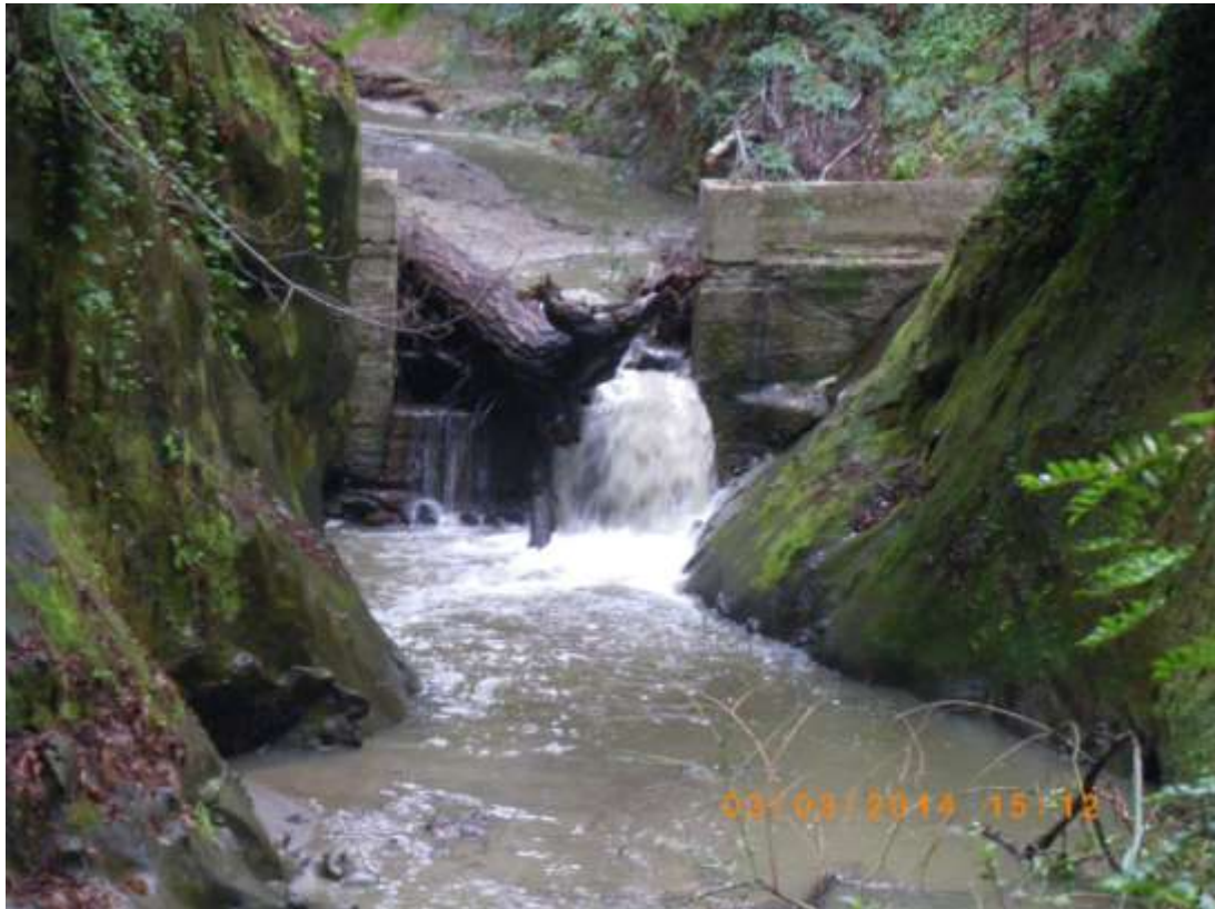
Flashboard dam on Bear Creek, downstream of Lanktree Bridge.
