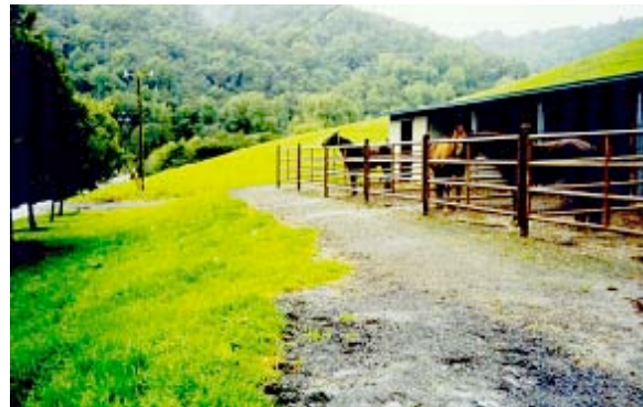
This filter strip is designed and maintained to transport a thin “sheet” of runoff slowly through vegetation. A gentle slope covered with lush vegetation achieves slow flow. Thick, sod-forming grass works best to trap sediment.
